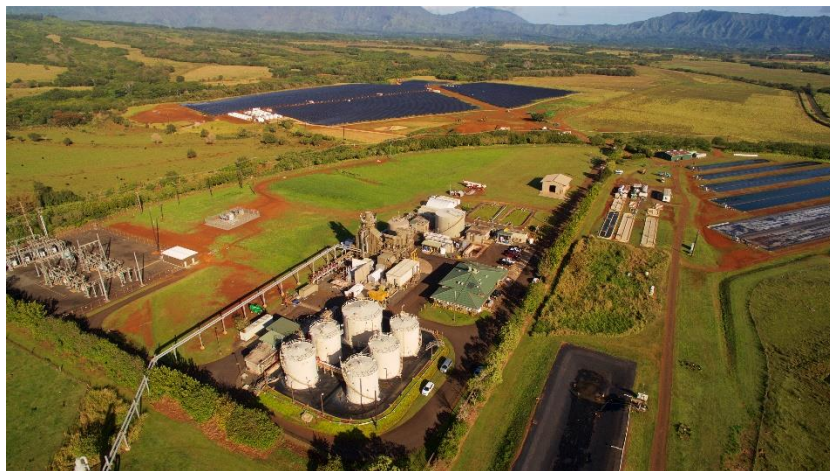
Photo caption: Aerial view of Kapaia Power Station and nearby Tesla solar storage facility
