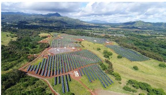
The AES Lāwa'i solar-plus-storage facility can provide up to 20 megawatts of direct-to-grid power during the day, along with five hours or 100 megawatt hours of electricity for use after sunset.
