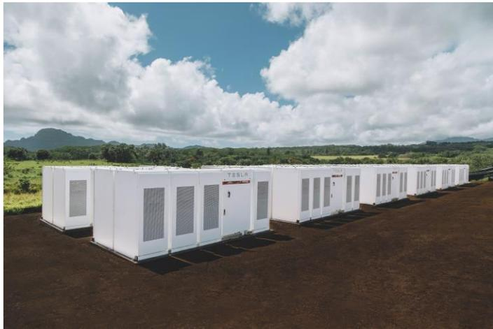
A total of 272 Tesla Powerpack lithium-ion batteries provide for 52 megawatt hours of solar dispatch during Kaua'i's evening peak
